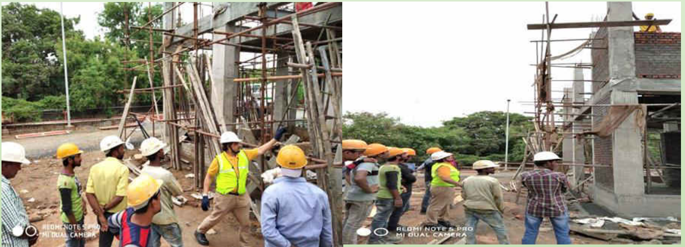
Practical demonstration in a construction site at the Leather Chemicals plant
